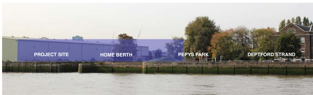
Project site viewed from river
