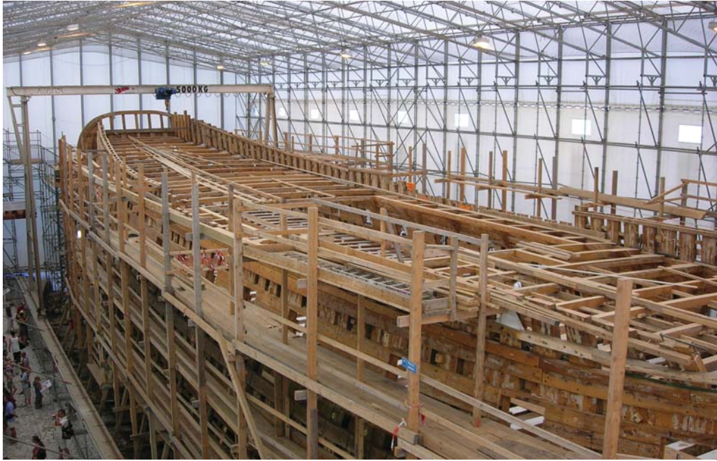
L'Hermione under construction showing enclosure
