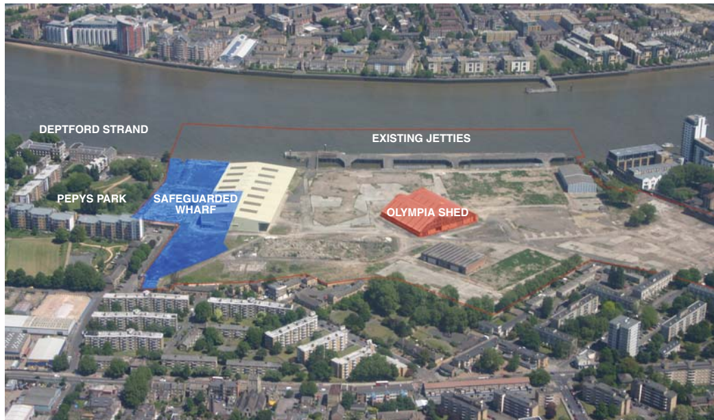
Convoys Wharf aerial photograph with location of Safeguarded Wharf and Olympia Shed highlighted
